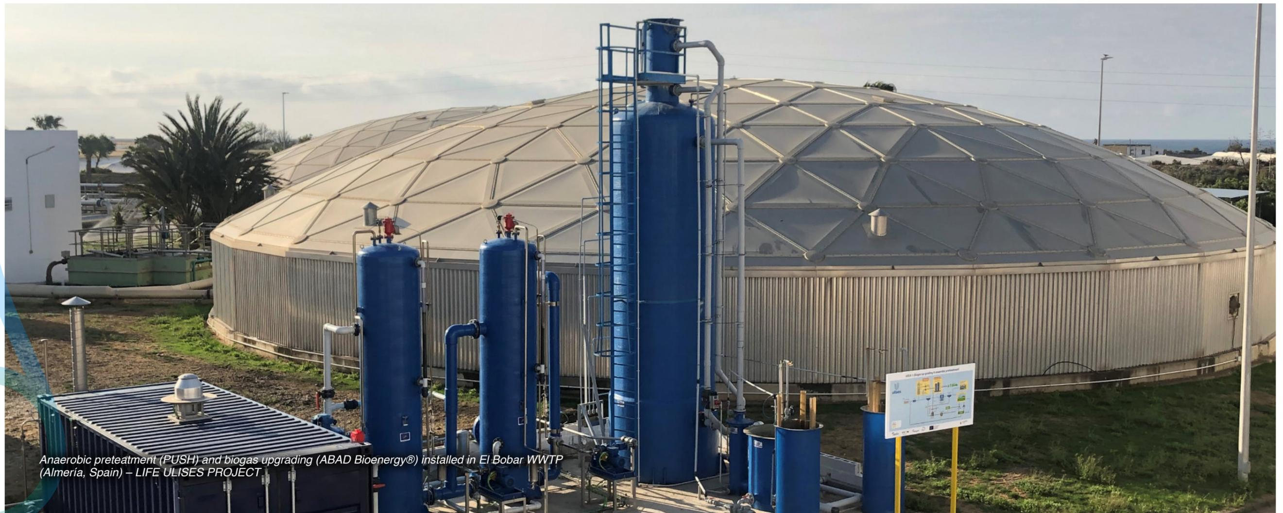
Anaerobic pretreatment (PUSH) and biogas upgrading (ABAD Bioenergy®) installed in El Bobar WWTP (Almería, Spain) – LIFE ULISES PROJECT
