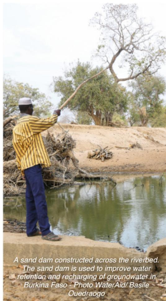
A sand dam constructed across the riverbed. The sand dam is used to improve water retention and recharging of groundwater in Burkina Faso - Photo WaterAid/ Basile Ouedraogo
